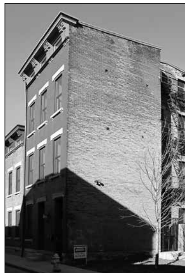
Fig. 11. Oblique view of 1420 Pleasant Street, Cincinnati, Ohio, showing south elevation windows and grocer's alley.
