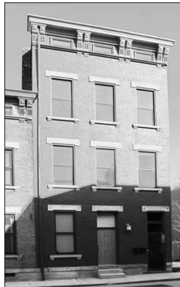
Fig. 10. View of 1420 Pleasant Street, Cincinnati, Ohio.
