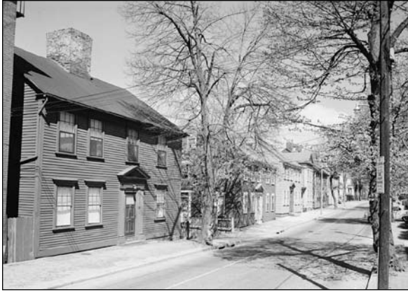
Fig. 6. Benefit Street on College Hill, Providence, Rhode Island, 1958 (Photograph by Laurence F. Tilley, HABS/HAER/HALS, Library of Congress) (HABS No. RI-148-2).
