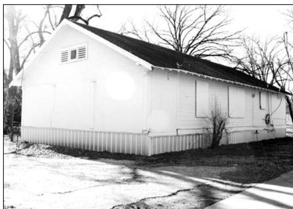
Fig. 11. The Lodge moved onto site during the 1930s, January 2010.
