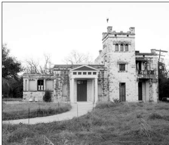
Fig. 10. Reconstructed driveway and new plantings, January 2011.
