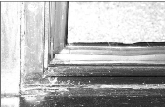
Fig. 14. Closeup of rust on interior face of frame, broken screws, and new gasket, 2008 (Photograph by Robert Whitehead).
