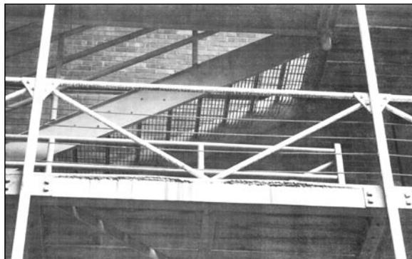
Fig. 8. Exit stair/pedestrian bridge with rusted perimeter, 2006 (Photograph by Baldwin White Architects).
