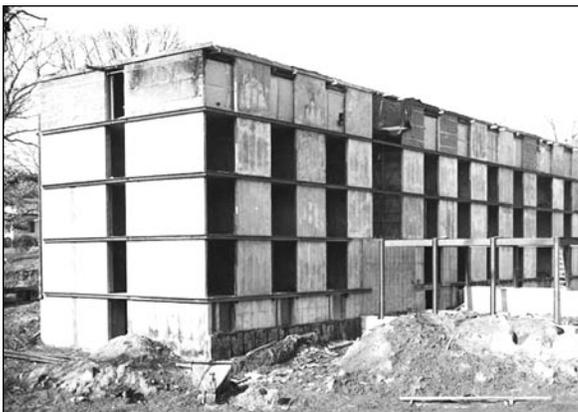
Fig. 6. Crawford Dormitories, 1953, Eero Saarinen & Associates. Dorm under construction showing precast assembly system (Presidential Files, Special Collections, Cowles Library, Drake University).
