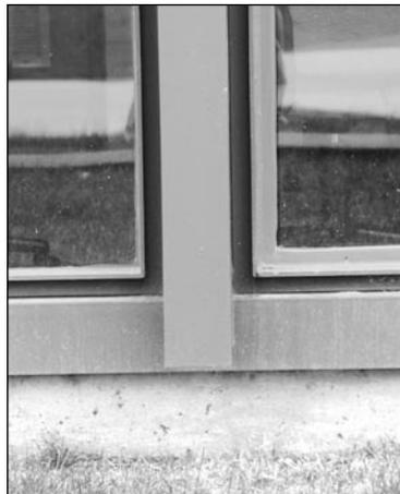
Fig. 15. Enlarged view of original and revised window jamb detail (painted rubber gas-keting), 2008 (Photograph by Robert Whitehead).
