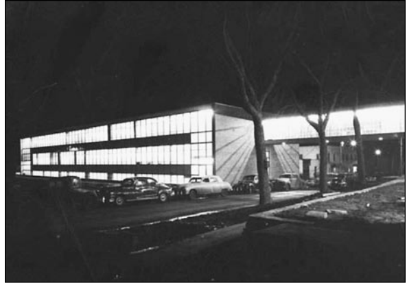
Fig. 2. Harvey Ingham Hall of Science, 1950, Saarinen, Swanson, and Saarinen. Nighttime view showing skywalk and curtain-wall system with metal panels (Harvey Ingham Hall of Science Photos Folder. Special Collections, Cowles Library, Drake University).
