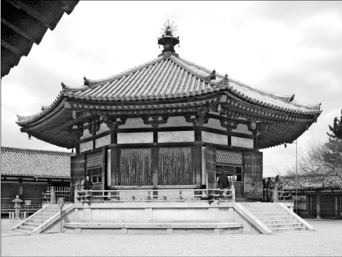
Fig. 1. The Yumedono at Hôryûji in 2006. Nara, Japan, built 739 (Photograph by Don Choi).
