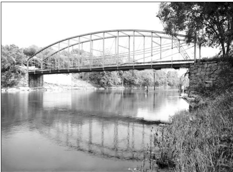
Fig. 1. Boardman's Lenticular Truss Bridge, Boardman's Road, New Milford, Connecticut, 1888, Berlin Iron Bridge Company, designer (Library of Congress, Prints and Photographs Division, Historic American Engineering Record, HAER CONN, 3-NEMI, 1-5).
