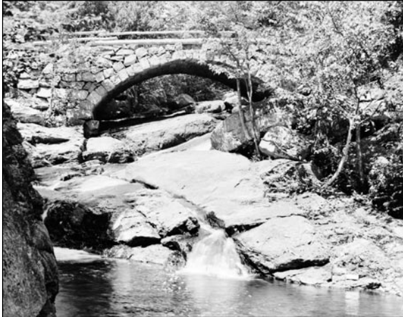
Fig. 3. Gleason Falls Dry-Laid Stone Arch Bridge, Beard Brook, Hillsborough, New Hampshire, mid-nineteenth century, designer unknown (Library of Congress, Prints and Photographs Division, Historic American Buildings Survey, HABS NH, 6-HILL.V, ID-2).
