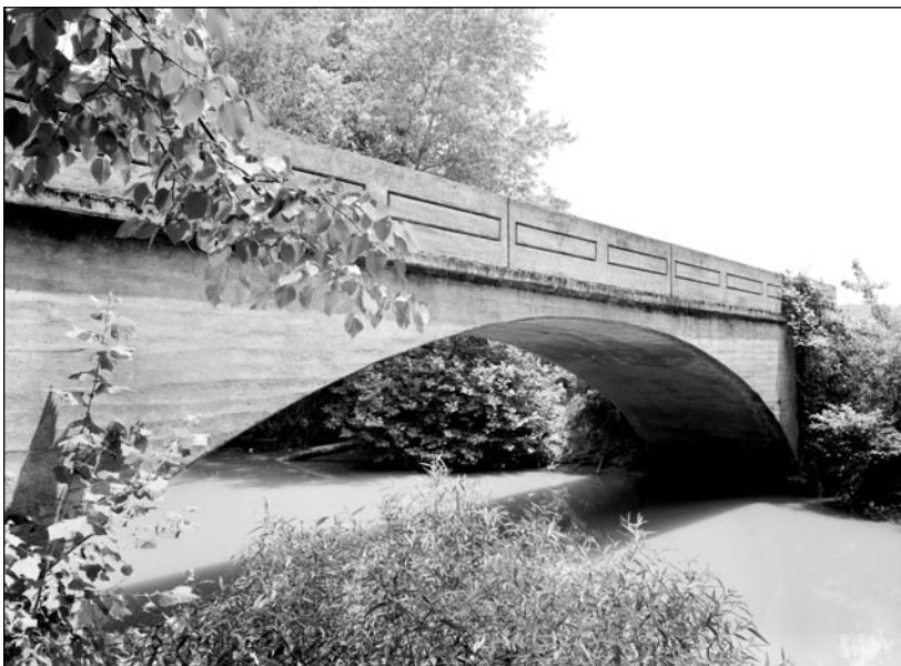
Fig. 5. Luten Bridge, County Road 228, spanning Pine Log Creek, Cash vicinity, Georgia, 1920, Daniel B. Luten Bridge Company, designer. The simple appearance of this concrete arch hides the fact that Luten was a pioneering innovator in reinforced concrete design (Library of Congress, Prints and Photographs Division, Historic American Engineering Record, HAER GA, 65-CASH.V, 1-1).
